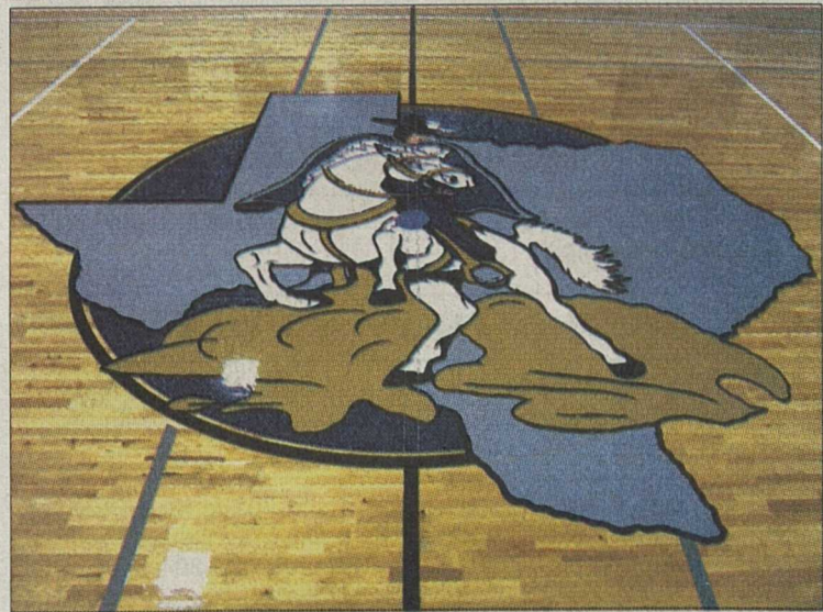
Work was recently completed on the new wood floor in Rice High School Gym. The project took about three weeks to complete and cost around $98,000.
